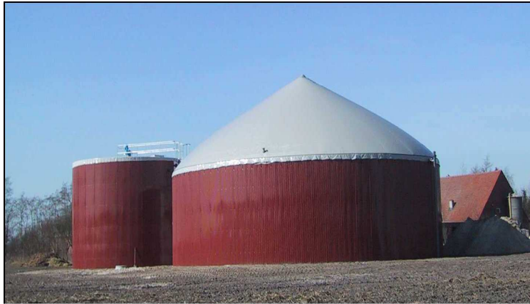
Fig.46. Installation de biogaz Schmits (Aschaffendorf)
