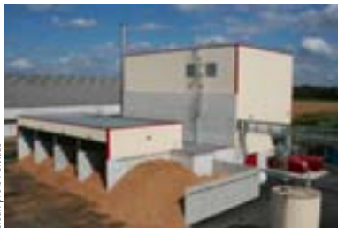
Chaufferie Biomasse Site Buchères
